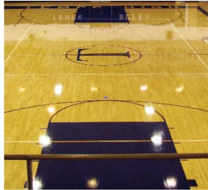
**WAXIE Ultra Sport** Premium Wood Coating is a single-component water-based coating. There is only a one hour dry time between coats under normal conditions. **WAXIE Ultra Sport** cures in just 24 hours, allowing the gym to be open for traffic the next day. The product's quick-prep, quick-dry and quick cure allow for wood floors to be recoated at anytime throughout the year.
